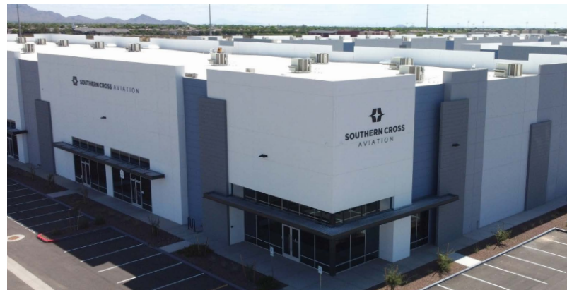
Southern Cross Mesa Warehouse
